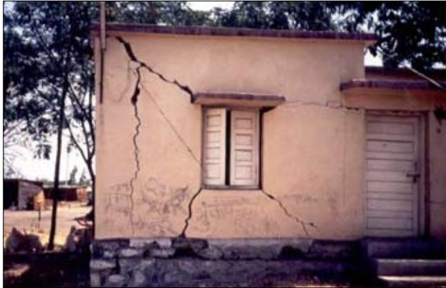
Figure 7: Shear cracks in an unreinforced brick masonry building from the 1993 Killari earthquake (WHE Report 21, India)
