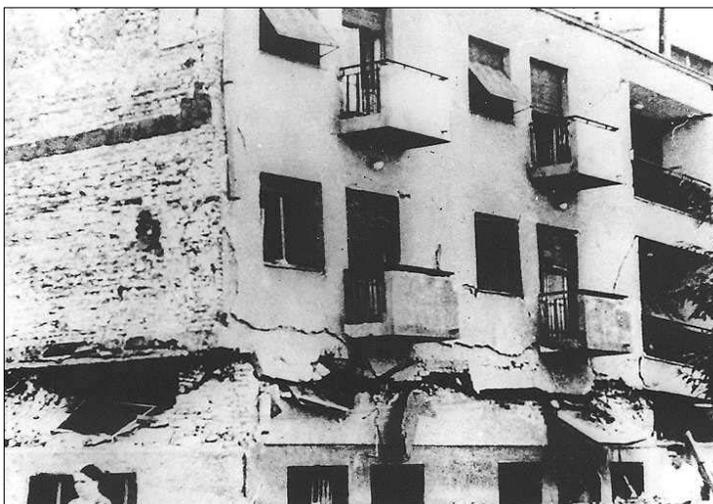
Figure 9: Severe damage to an unreinforced brick masonry building due to inadequate wall density in the 1963 Skopje, Macedonia earthquake (WHE Report 73, Slovenia)
