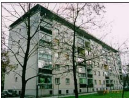
Figure 4: Six-story unreinforced brick masonry apartment building (WHE Report 73, Slovenia)
