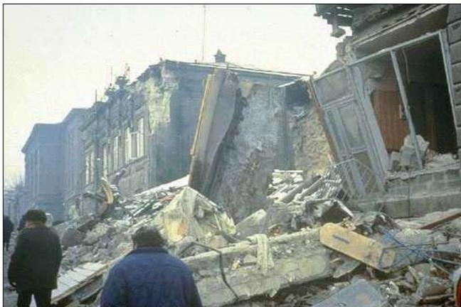
Figure 8: Collapse of brick masonry buildings in the 1988 Spitak earthquake (WHE Report 4, Armenia)
