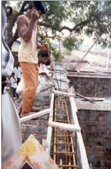
Figure 10: Construction of a RC ring beam/lintel band (WHE Report 21, India)
