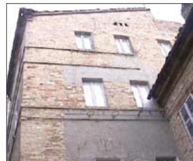
Figure 5: Four-story building with strengthened spandrels in Offida (WHE Report 29, Italy)
