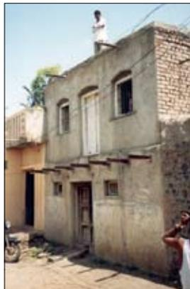
Figure 3: Unreinforced brick masonry building with reinforced concrete roof slab (WHE Report 21, India)
