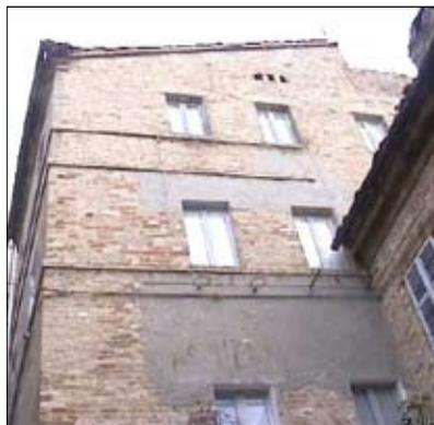
Figure 11: Grouting to improve capacity of spandrel walls (WHE Report 29, Italy)
