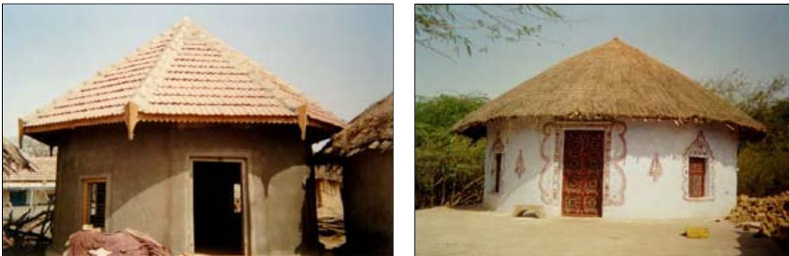
Figure 2: Earthquake-resistant bhonga houses in India: traditional thatched roof (left) and modern clay tile roof (right) (WHE Report 72)
