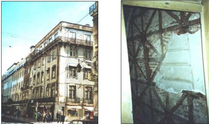
Figure 5: The exterior of a Pombalino building (left) and details of timber bracing (right) (WHE Report 92, Portugal)
